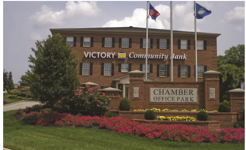
Front view of building
